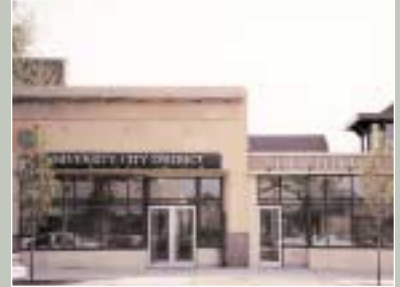
University City District Operations Center at 40th & Chestnut streets.
