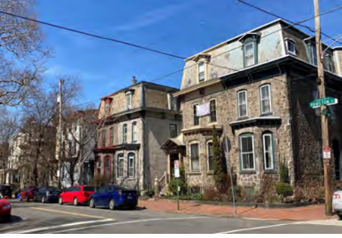
Figure 2 - 3500 Hamilton Street North
