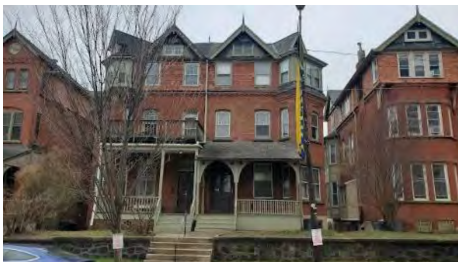
Figure 36. 3316 Arch Street is one of a row of 1880 twin residences designed by architect Albert W. Dilks in 1880 and now owned by Drexel University.
