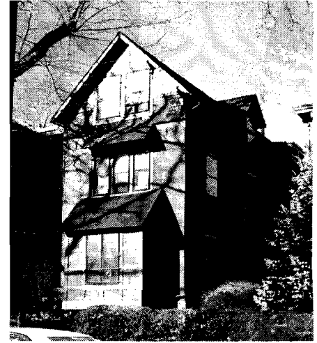
3309 Baring Street, home of the Monaghans (Doug Ewbank)
