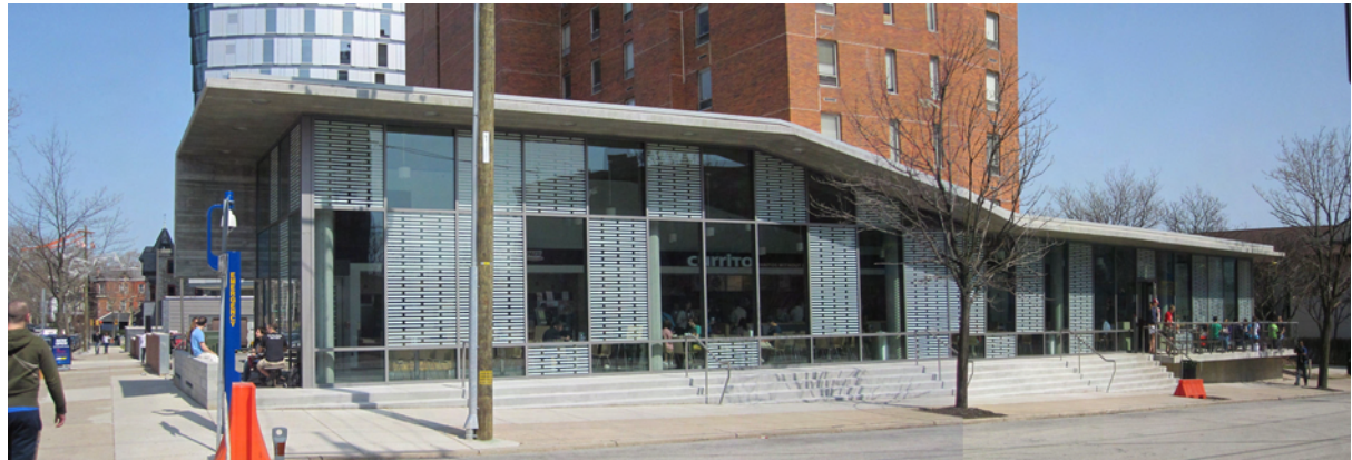
The new dining terrace at 34th and Race Streets is open to both residents and students.
