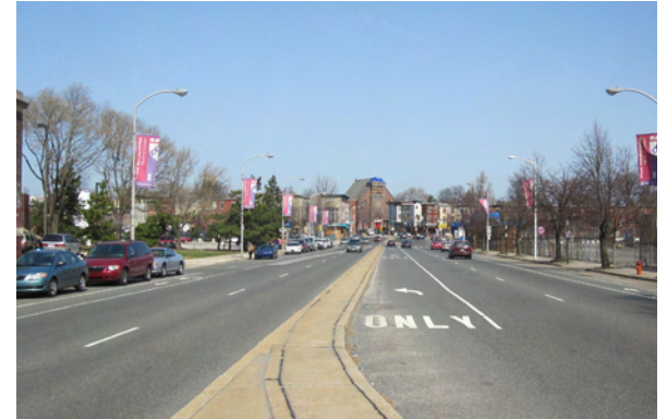
A barren median and an over-wide 38th Street.
