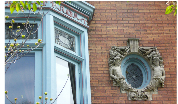
Historic details contribute to Powelton Village's historic designation.
